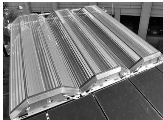
**FIGURE 1.** Detailed view of the MCT system installed alongside a conventional PV system on the same mounting support.
