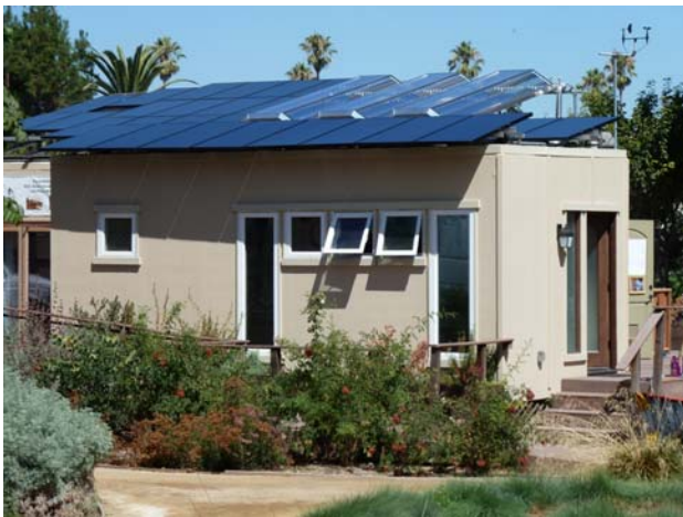
Fig. 2: A CPV-T ANU-Chromasun Micro-concentrator on a rooftop installation integrated with conventional PV panels at the Santa Clara University 2009 Solar Decathlon House.
